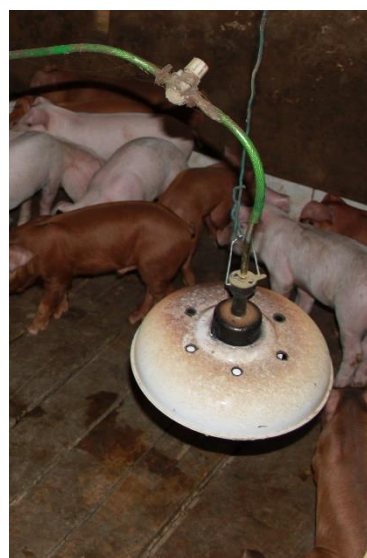
Picture 4-2: a) Simple self-made flaring system in Nam Dinh. b) Heating lamp for piglets running on biogas in Phu Tho.
