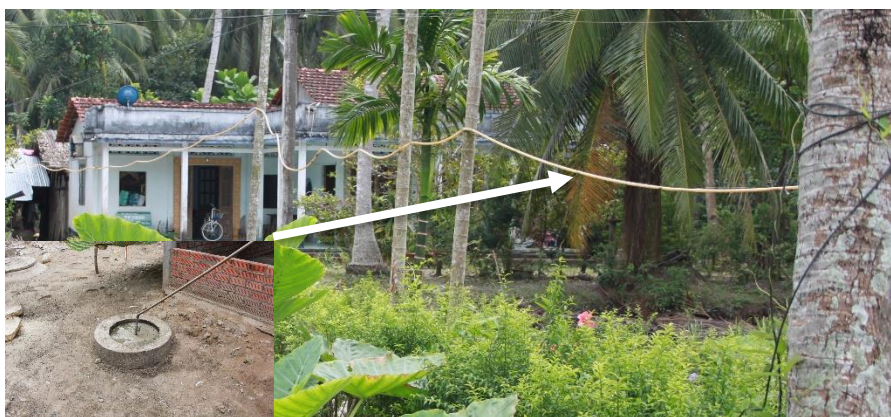
Picture 4-1: Gas pipe connecting 20 households from a farm with 450 pigs in Ben Tre
