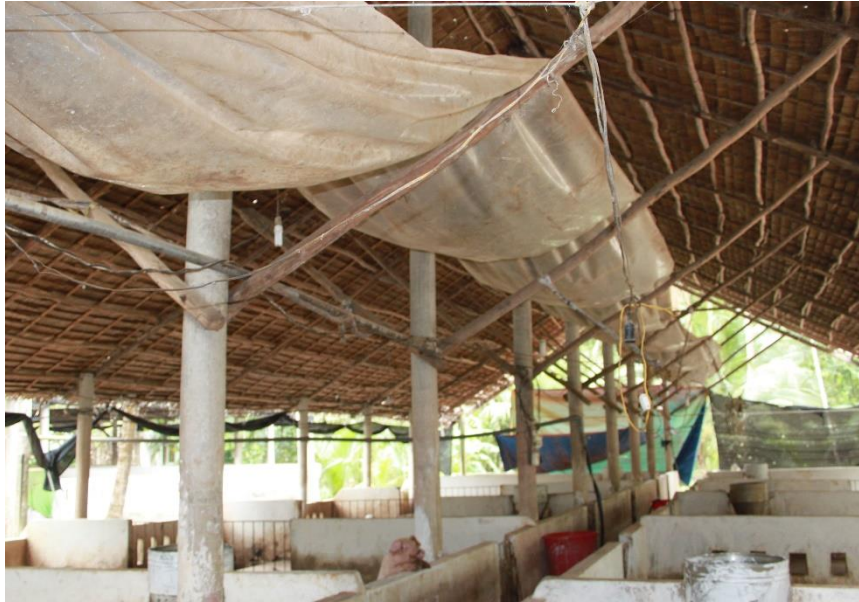
Picture 4-3: Simple gas storage system mounted under the roof.
