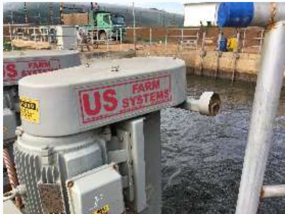
Wastewater cleaning system
