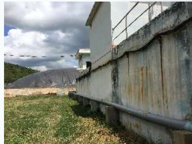
Wastewater going to the biogas
